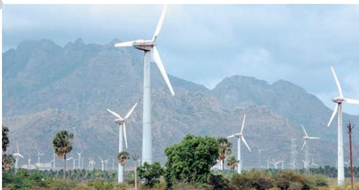
The electrical generators used on wind turbines in sites like Muppandal, produce an output AC of 240 V and a frequency of 50 Hz even when the wind speed is fluctuating. A
